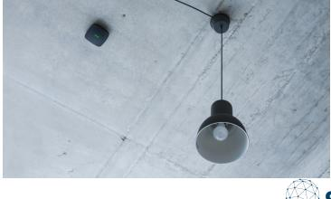
The device detects smoke through a camera with a photoelectric sensor. An added chemical element detects carbon monoxide and raises the alarm.
